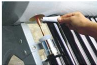
Daub thermal grease on heat pipe condenser
